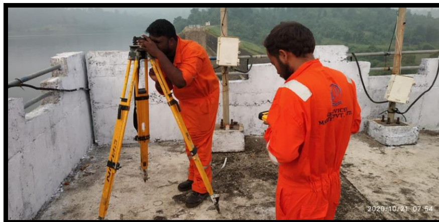
RTK Base Set up At Dam
